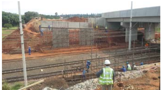
West pier construction – pier and abutment wall construction is ongoing.
