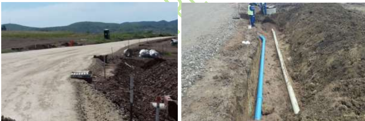
Figure xx: Empangeni Mega Housing project G5 Layer completed and Water & Sewer Pipes Reticulation
