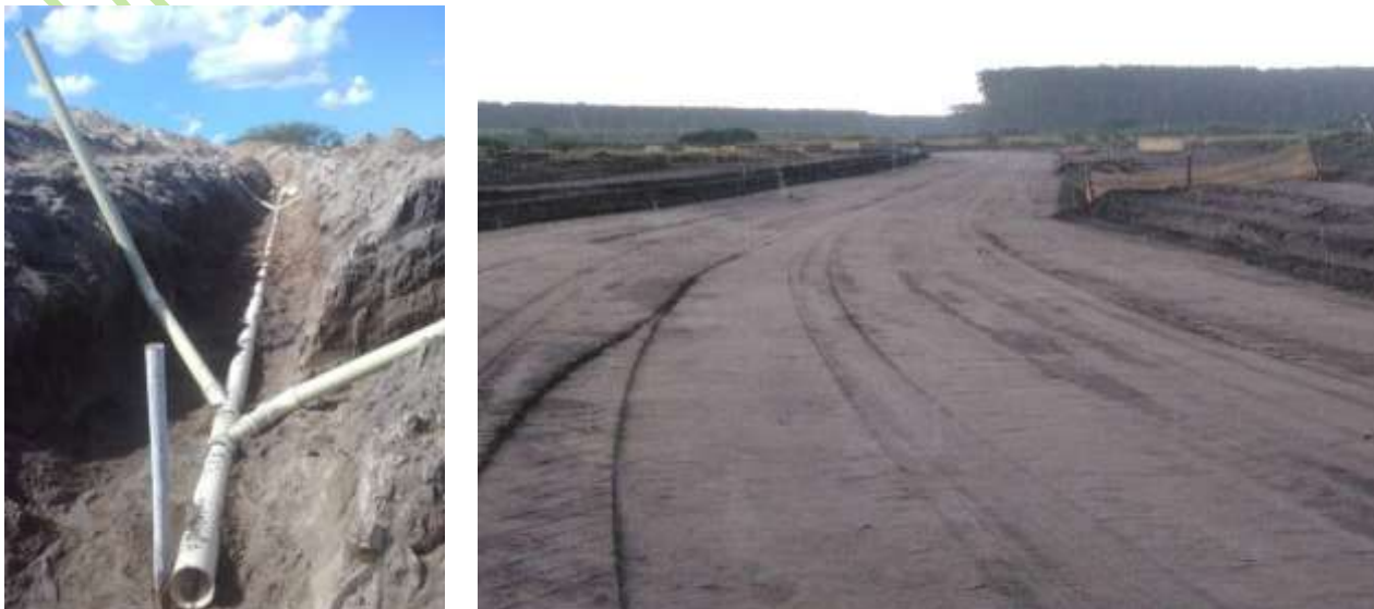
Figure xx: Aquadene Housing Project sewer pipe reticulation underway and roadworks
