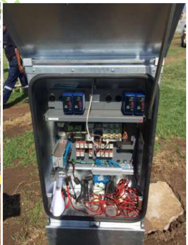
Replacement and upgrade of Traffic signal controllers in Empangeni
