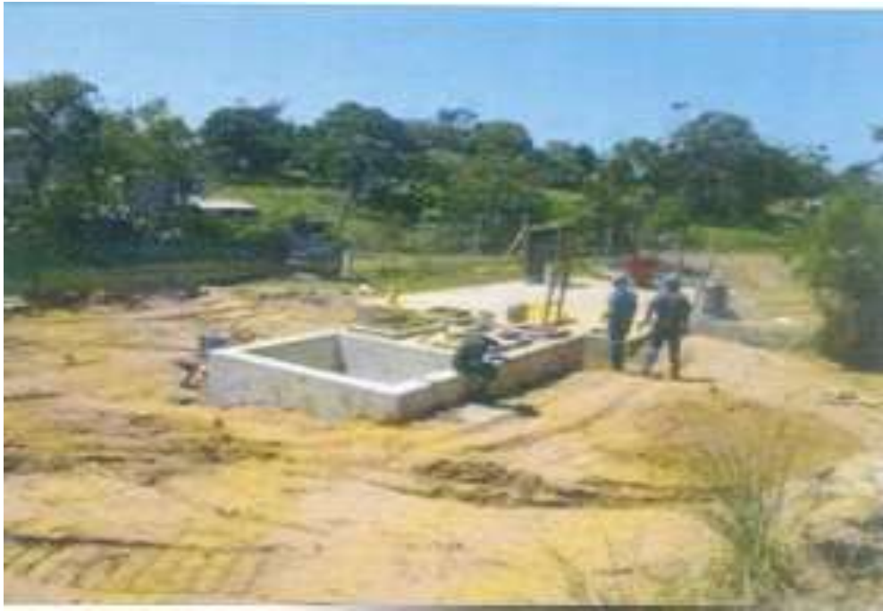
Mandlazini Sewer Phase 2A – Pump station construction
