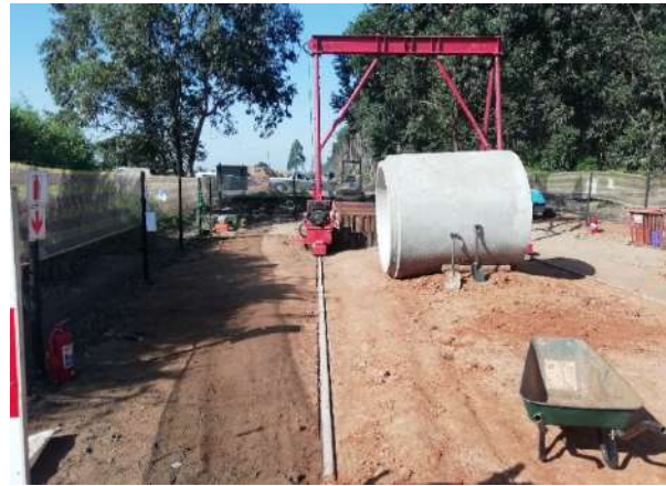
Construction of Outfall Storm water pipe and canal – Open Cut for pipes
