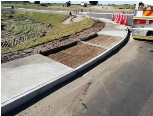
Construction of Access intersection - Storm water canal and walkways
