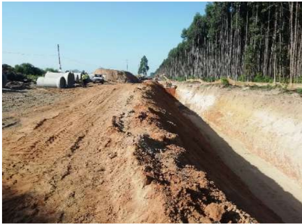
Construction of Outfall Storm water pipe and canal – Open Cut for pipes
