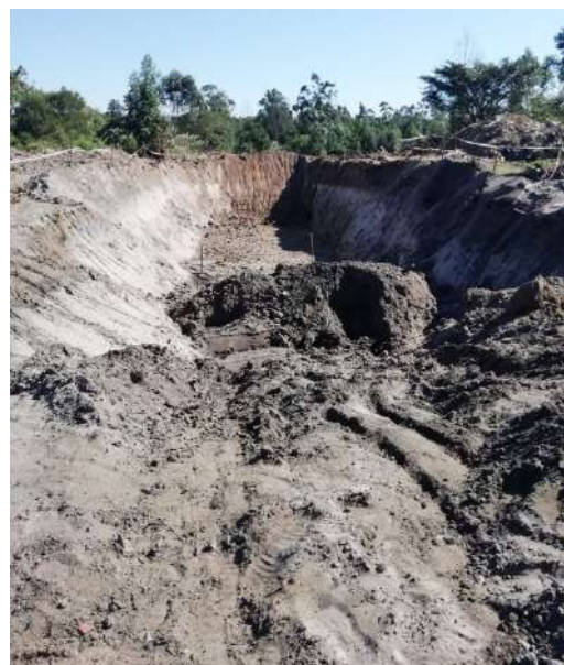
Construction of Outfall Storm water pipe and canal – Open Canal
