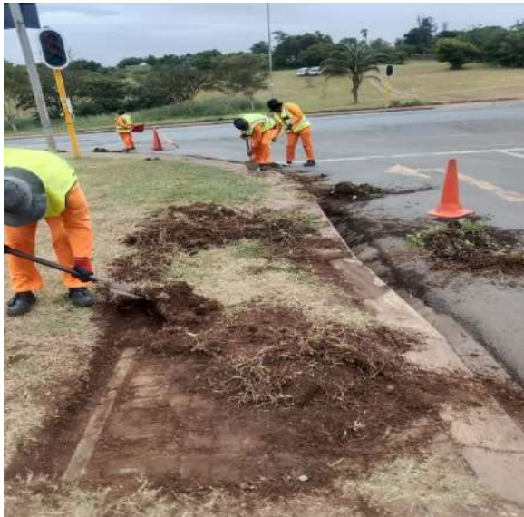
Empangeni: Cleaning of Storm-water drainage – R34 Empangeni CBD
