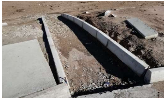
Construction of Access intersection - Storm water canal and walkways
