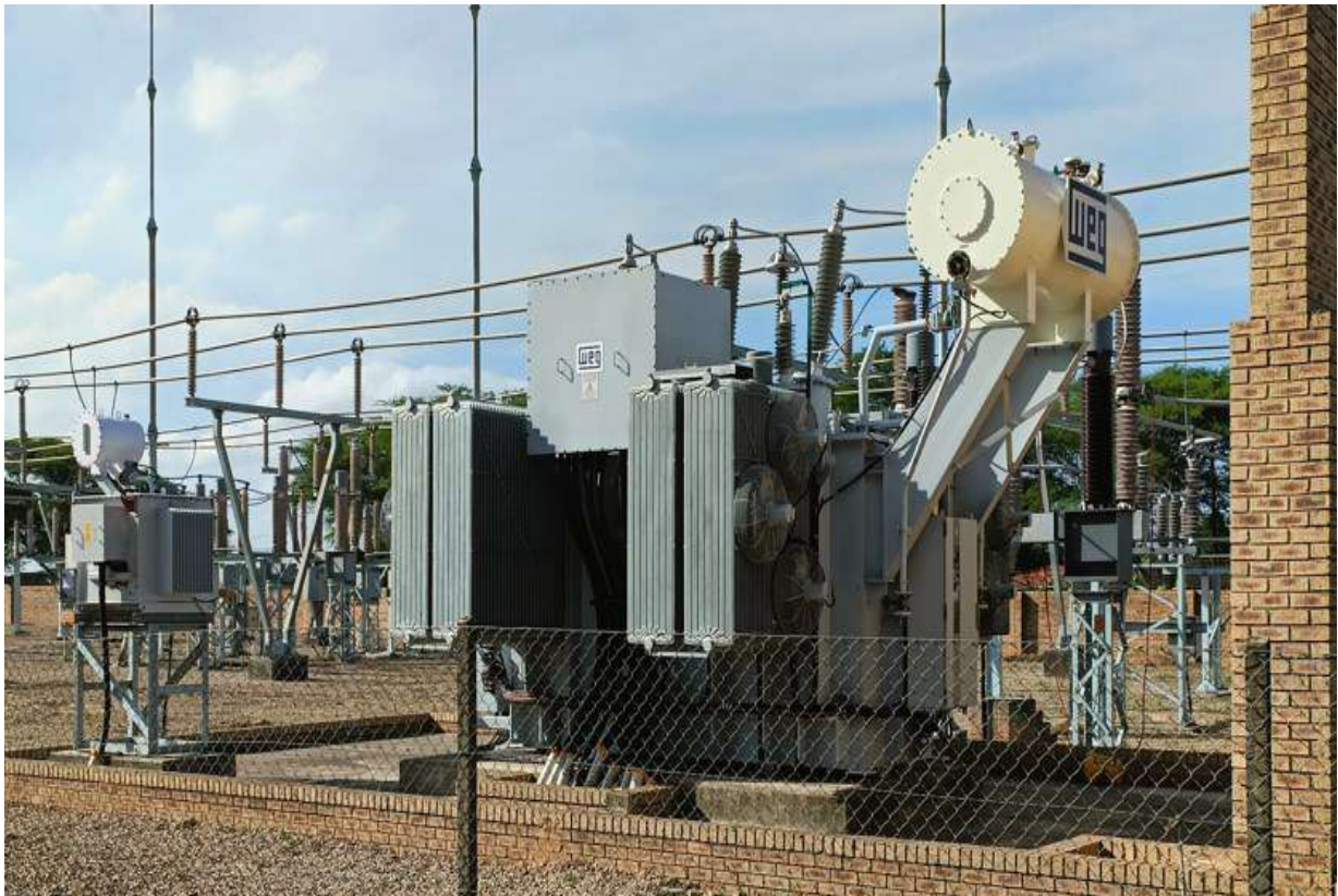
Cygnus Substation 132/11kV 40MVA transformer installation: Ward 22; Co-ordinates: 28°53'09.0"S 31°54'02.5"E
