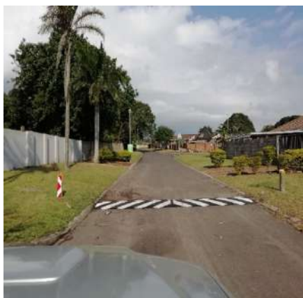
Speed humps Constructed in Birdswood – Drongo Domain Road
