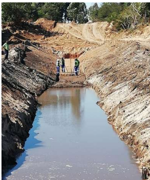
Construction of Outfall Storm water pipe and canal – Open Canal
