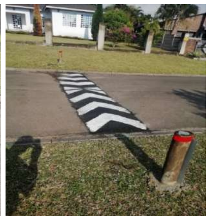
Speed humps Constructed in Birdswood – Drongo Domain Road
