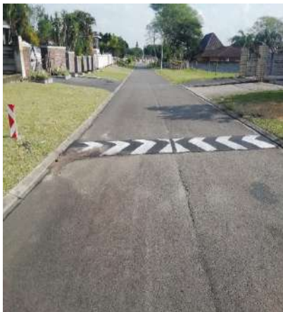
Speed humps Constructed in Mandlazini Airport Road
