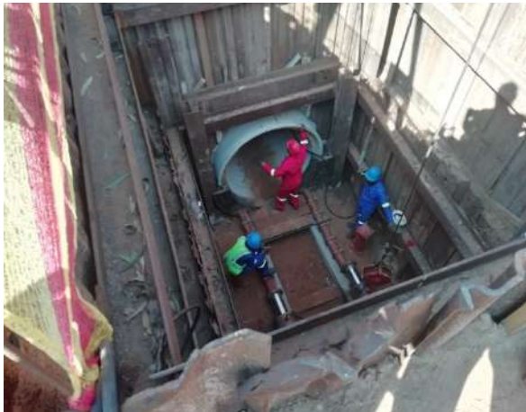
Construction of Outfall Storm water pipe and canal – Pipe Jacking Pit
