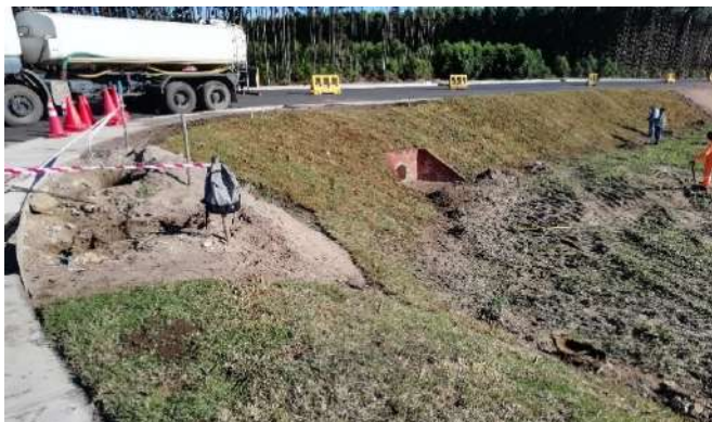
Construction of Access intersection - Storm water canal and walkways
