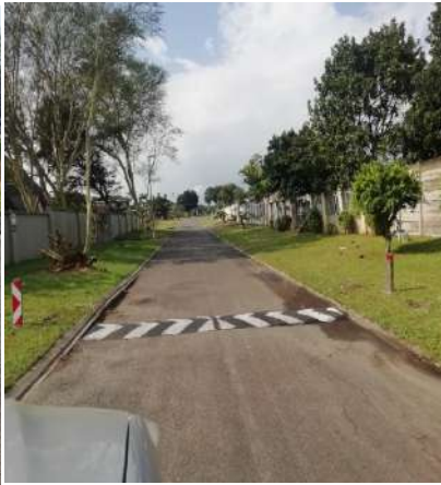
Speed humps Constructed in Mandlazini Airport Road
