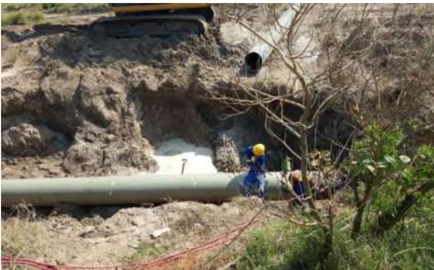
Figure 51: Pipe repairs
