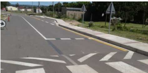
Road markings, painted pedestrian crossing, signage and bus/taxi layby:
