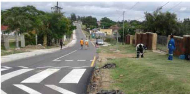
Municipal standard Concrete walkways with the red brick strip were constructed.
