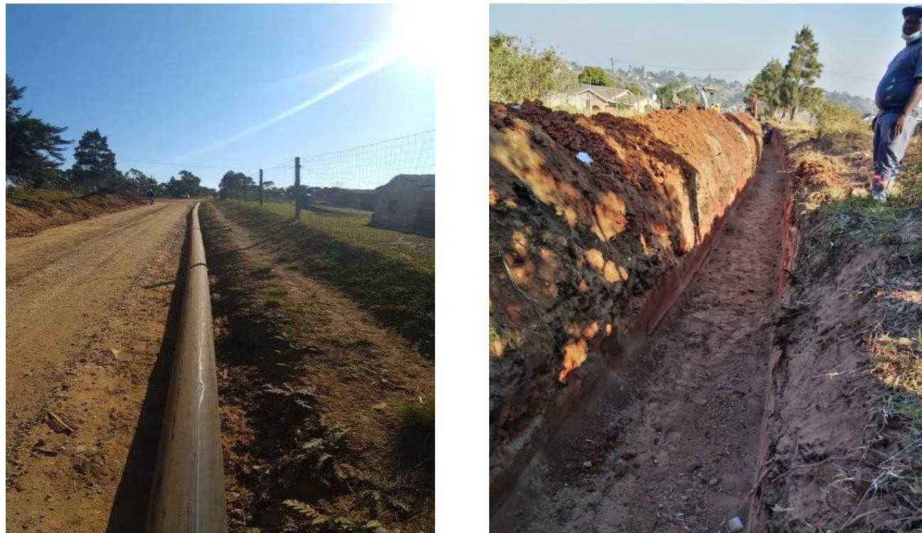
Figure 155: Construction Of Bulk Pipeline From Vulindlela Reservoir To Reservoir B & C
