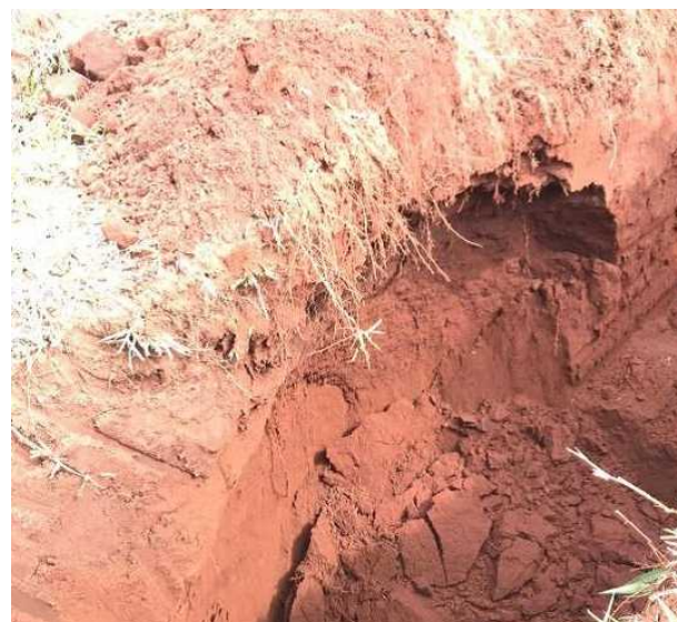
Collapsing side wall of excavation for in-situ Line
