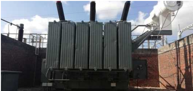
Figure 246: Refurbished 132/11kV 30MVA transformers at Hercules Substation: Ward 1; Co-ordinates: 28°44'58.4"S 32°02'40.7"E
