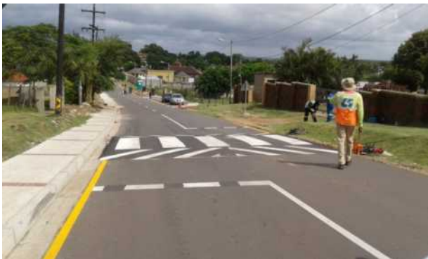
Traffic calming measures installed i.e. speed humps at dedicated pedestrian crossings:
