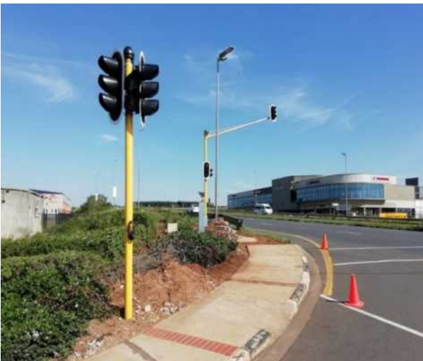
Installation of new Traffic Signals at John Ross / Eco Park intersection:
