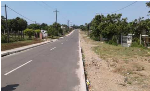
The completed Bus Road that was under construction, with a kerb and walkway on the one side and an edge beam on the other.
