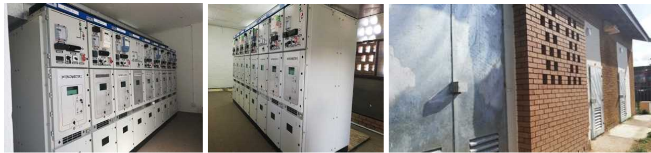
Figure 167: Formalhaut Switching Station: Replacement of MV Switchgears and refurbishment of MV switch room: Ward 1; Co-ordinates: 28°46'53.0"S 32°06'04.2"E
