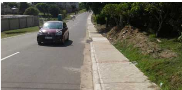
Walkway, kerbs, premix surface and line markings with a stormwater kerb inlet.
