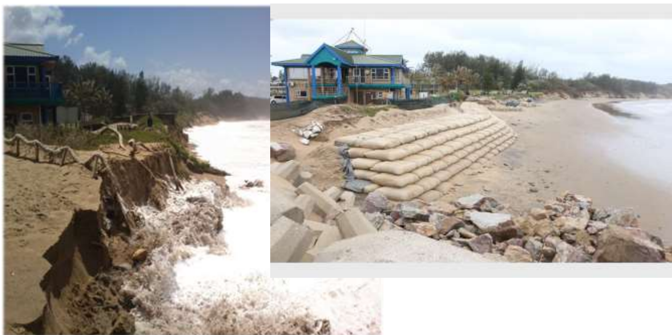
Figure 22: Coastal Erosion and Installed Defenses
